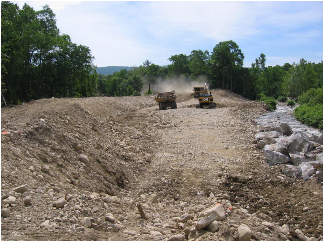
Roaring Branch, Bennington, 2010 Removal of confining berm and restoration of flood plain
